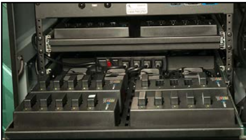
Figure 52: 5-Bay Battery Chargers
