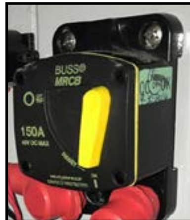
Figure 25: Battery Breaker (On Position)
